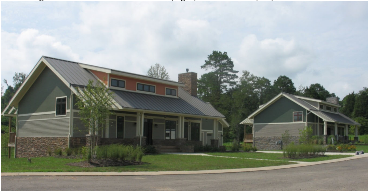
Figure 1. Front View of House 1 (right) and House 2 (left) from the Street
