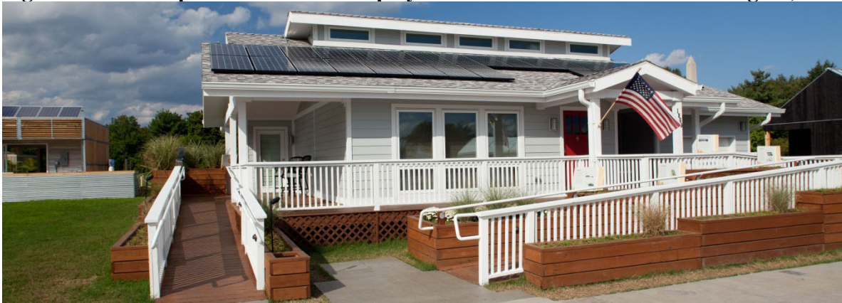
Figure 1. The 2 nd place INhome on display at West Potomac Park in Washington, D.C.
