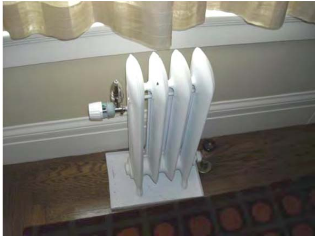
Figure 8. One-Pipe Low-Pressure Steam Thermostatic Radiator Valve (TRV)
