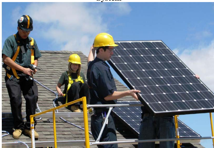
Figure 4. E.C. Goodwin Technical High School Students Installing Solar Photovoltaic System
