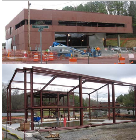
Figure 3. MAXLAB and FRPs Under Construction
