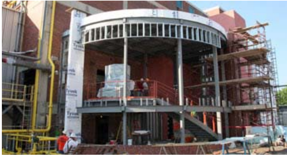
Figure 8. Biomass Steam Generation Plant Under Construction
