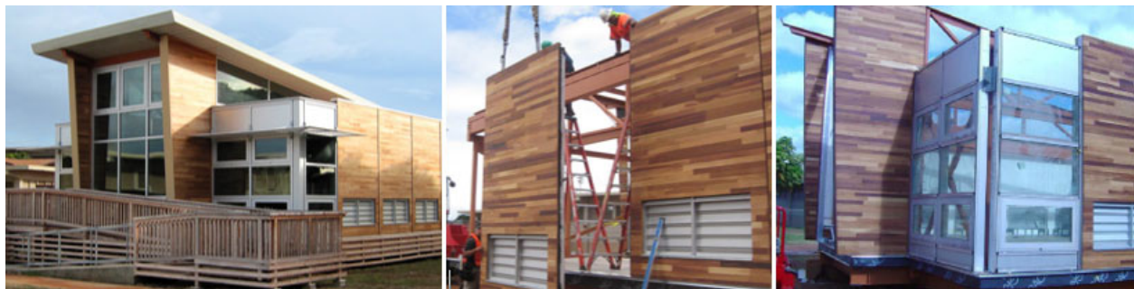
Figure 1. Project Frog Ilima Int. School, Ewa Beach, Hawaii. Finished bldg. (left), wall panels (center), window components (right).
