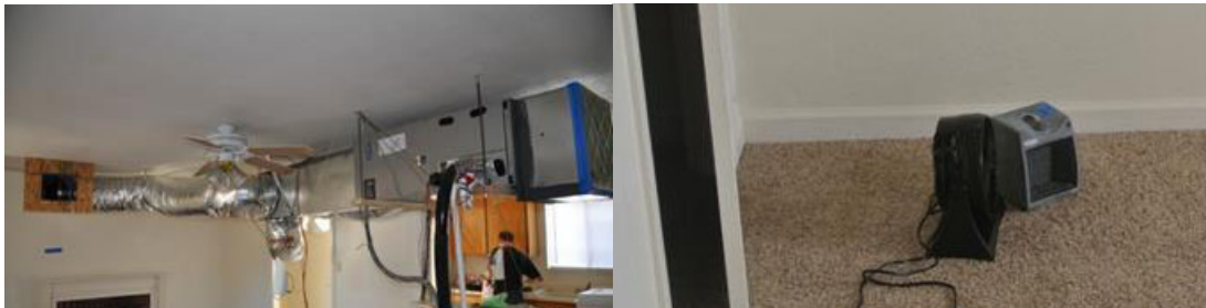
Figure 1. Reference "yardstick" air conditioner cooling system and room-by-room electric resistance heating system. Source: R. Chitwood, pers. comm., 2012.
