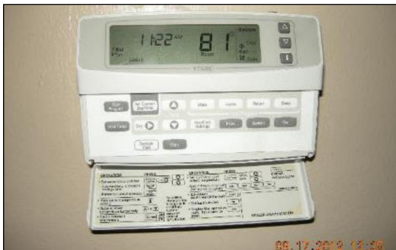
Figure 3: Site 28 existing thermostat, a Trane XT500C programmable model.
