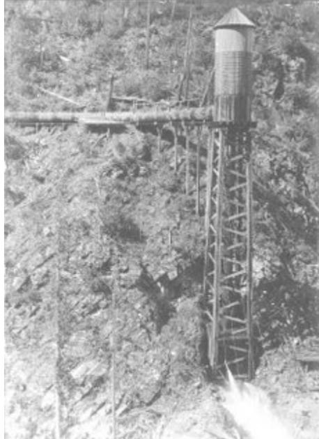
Figure 1. The HAC constructed at Ainsworth, British Columbia in 1898, with air power rating of 431kW, utilizing head of ~33 m head, ~1.9 m<sup>3</sup>/s water and producing 2.2 Sm<sup>3</sup>/s (4667 Scfm) air at 6 bar gauge (Pavese, Millar and Verda 2016). This HAC is reported to have provided air to the Kaslo Copper Mine, 2 to 3 miles away from the installation (H 2016).
