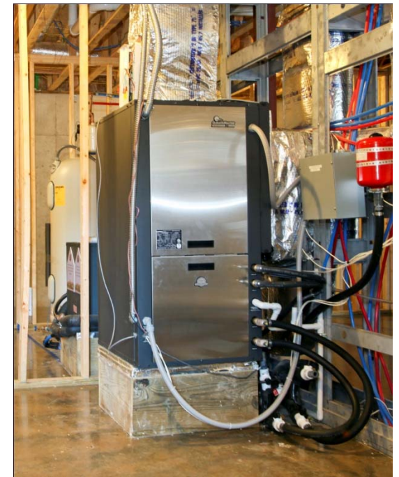
Single Unit [Water Heating; Heating/Cooling]
