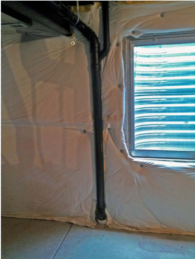
Replace section of drain
