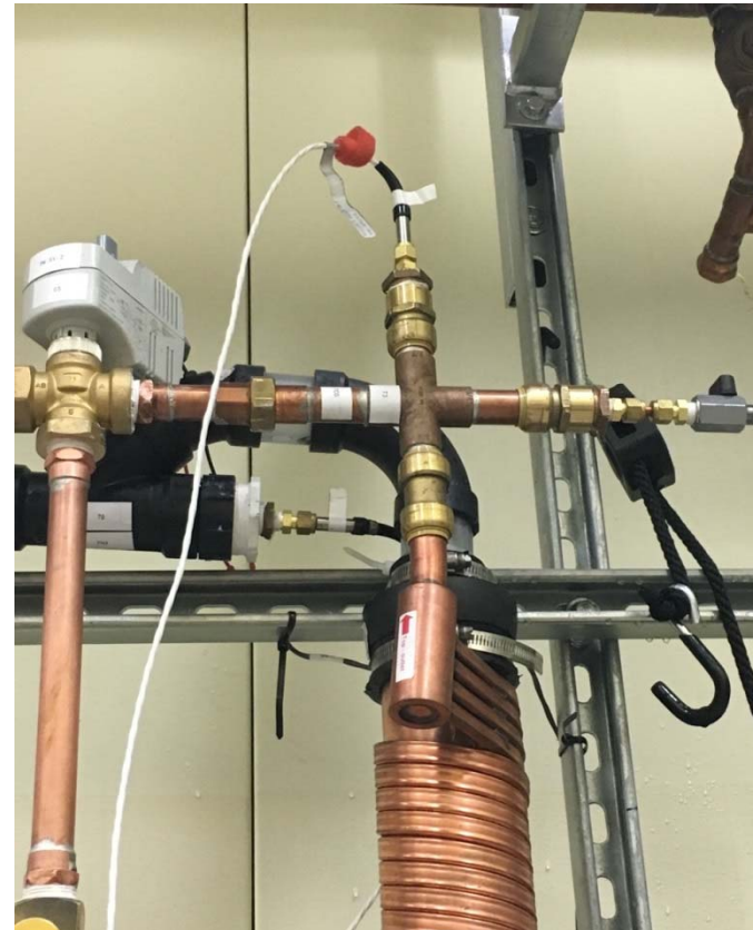
Cold Side Outlet/Drain Side Inlet
