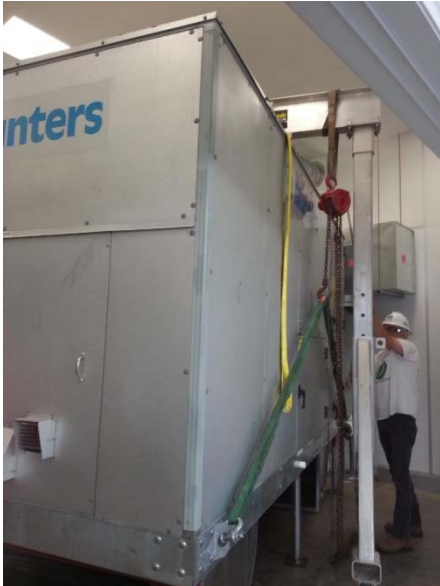
End use Equipment Testing
