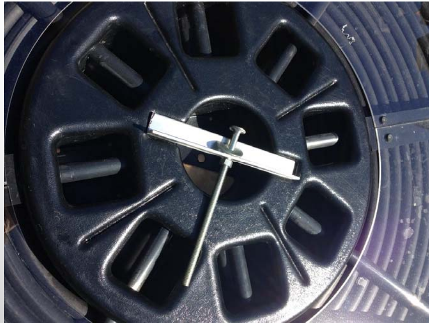
one bolt collector
