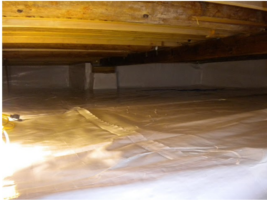
Existing · Crawl Space
