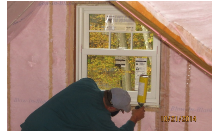
Air sealing during construction
