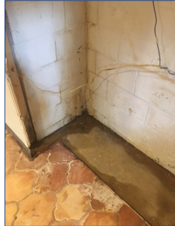
Seepage After 3" Rain Deluge
