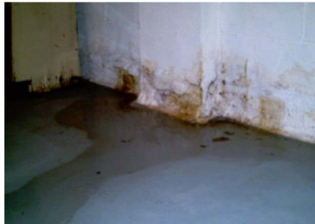
Water damage in the basement.
