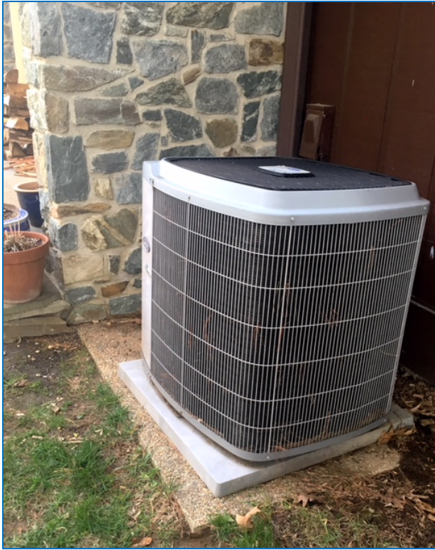
Heat Pump Slab Sloped Toward Corner
