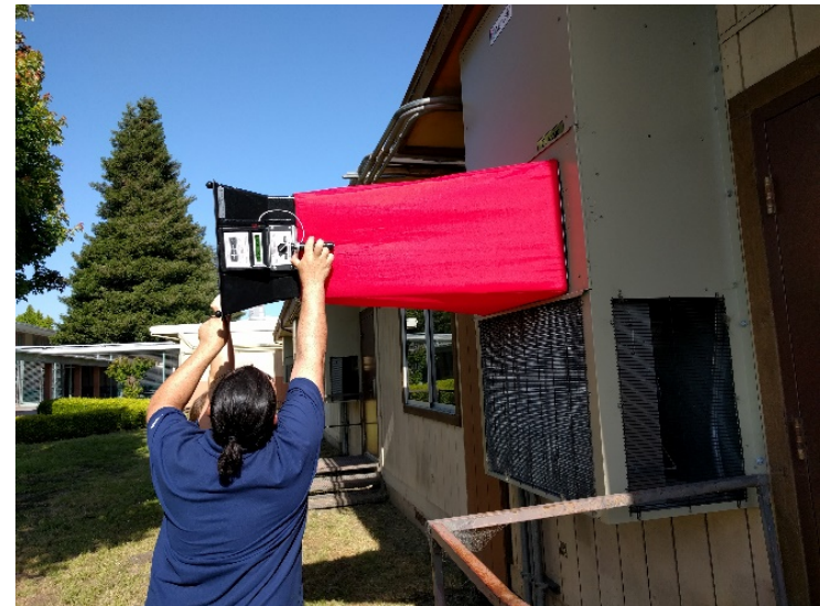
Flow capture hood to measure outdoor air rate
