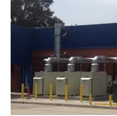
Combined Heat and Power
