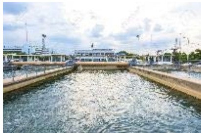
WATER TREATMENT (WTP)
