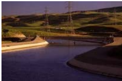
SOURCE WATER PUMPING (WSO)
