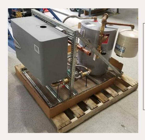
72 kW Electric Tankless 20 Gal Storage Tank circulator, aquastat, valves, etc.
