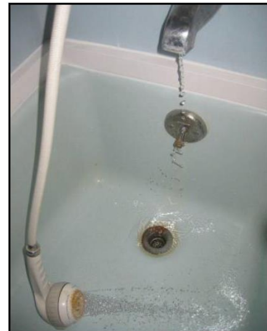
Taitem Engineering, PC, 2011. “Leaking Shower Diverters”
