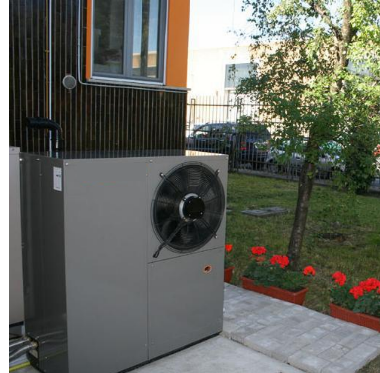
GAHPs commercially available in EU for home heating, in 2016 an 18 kW (61 MBH) output released by Italian mfr. Unit costs are prohibitive for US, > $11,000 (excl. shipment)
