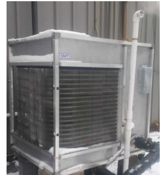
Heating-only 80kBtu/hr unit operating in 2016
