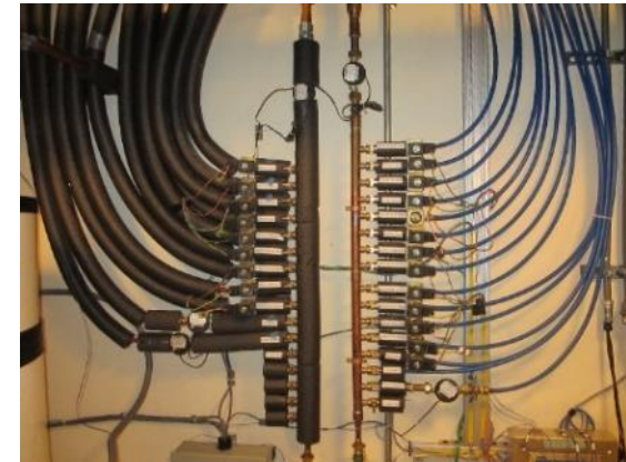
PEX lengths from manifold to fixture
