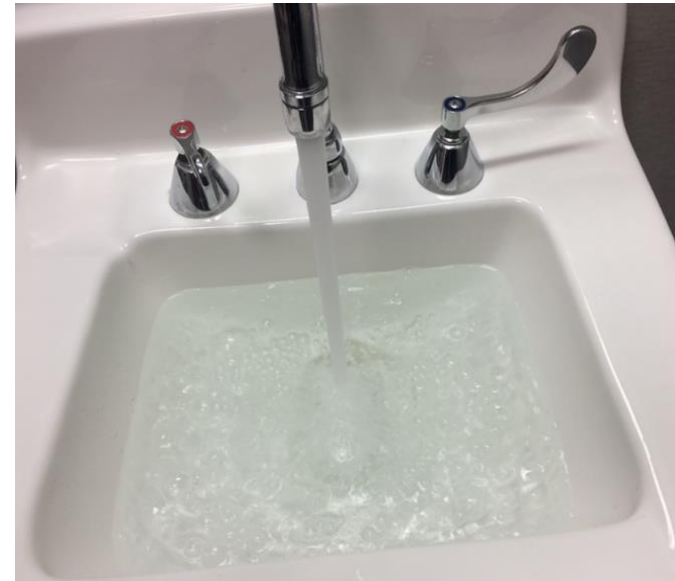
2016: Detroit Water with Corrosion Control
