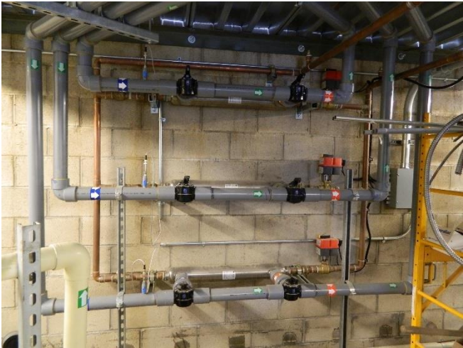
CHP heat exchangers
