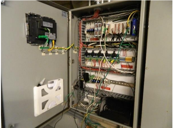
Controller and Data communication center
