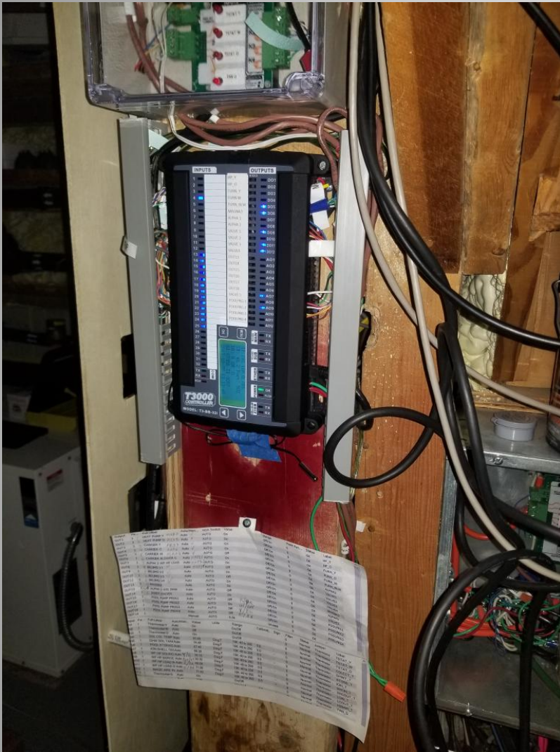
TEMCO T3 DDC SYSTEM CONTROLLER
