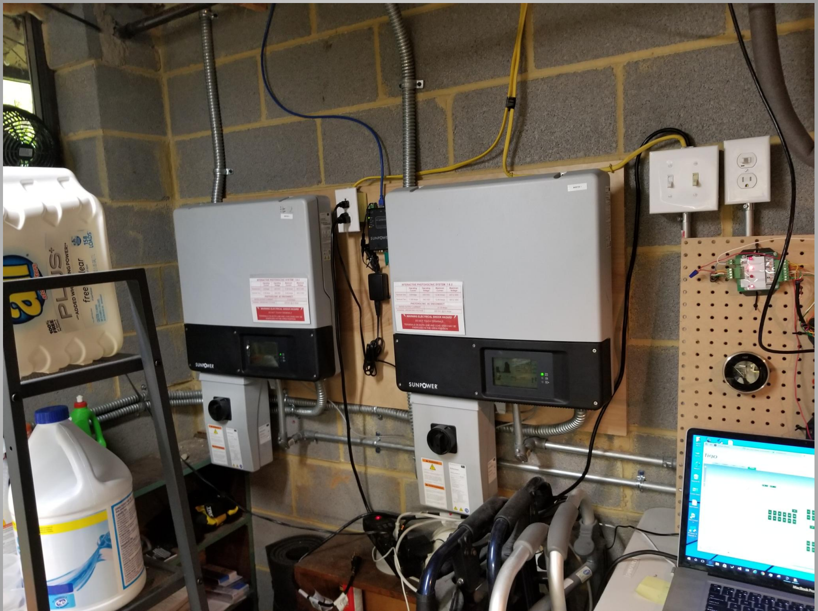
TWO SUNPOWER/SMA-AMERICA 5 KW PV INVERTERS WITH EMERGENCY POWER OUTLET ON RIGHT
