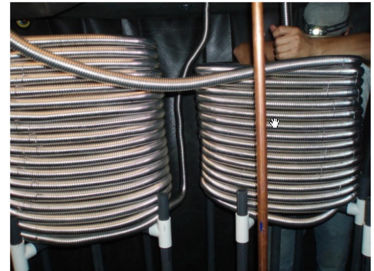
Heat Exchangers 304 SS 1" Dia. x 100ft each Corrugated, immersed
