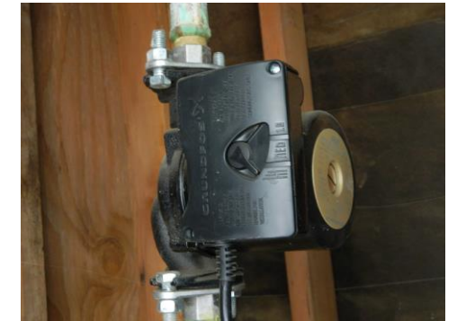
Hot water circulator
