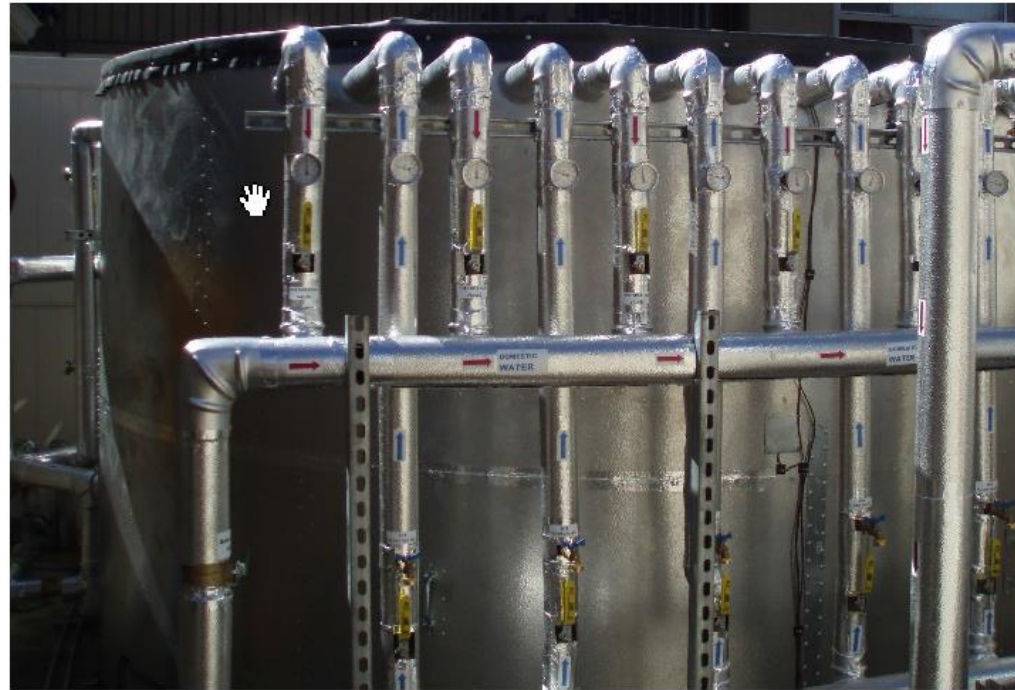
Heat Exchanger with Temperature Gages
