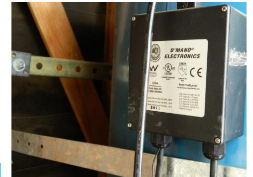
Aquastat for hot water temperature setting & sequencing
