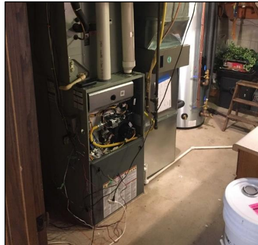
Hydronic A-Coil and Furnace (Blower)
