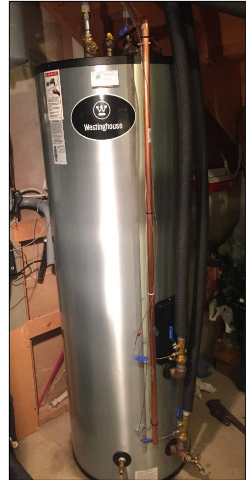
Indirect DHW Tank
