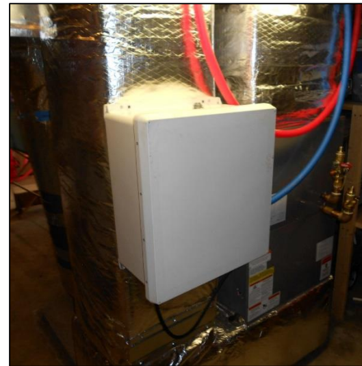
Hydronic Air Handler with Internal Pump
