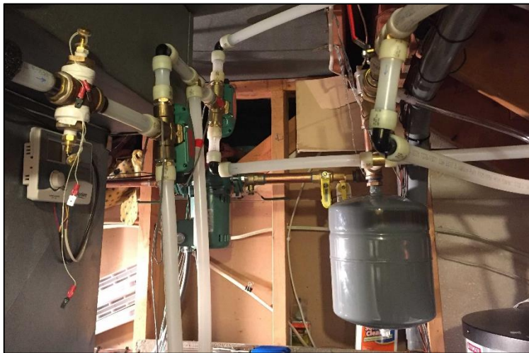
Main Loop Circulating Pump and 3-way valves
