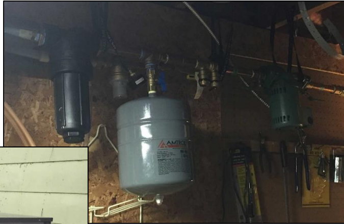
Main Loop Circulating Pump
