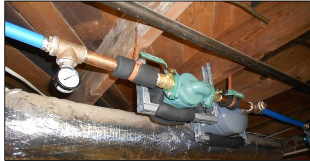
Main Loop Circulating Pump
