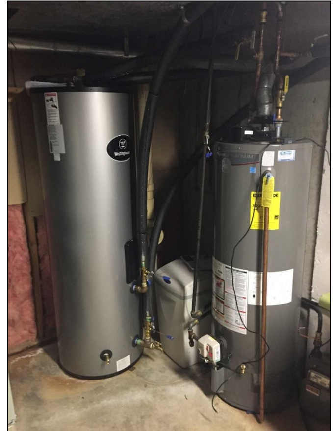
Indirect DHW Tank & Standard Gas WH
