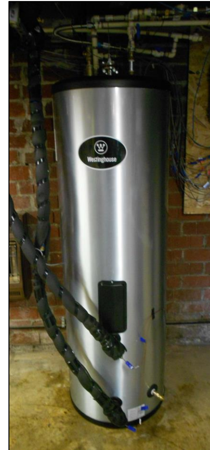
Indirect DHW Tank (Tank #2)
