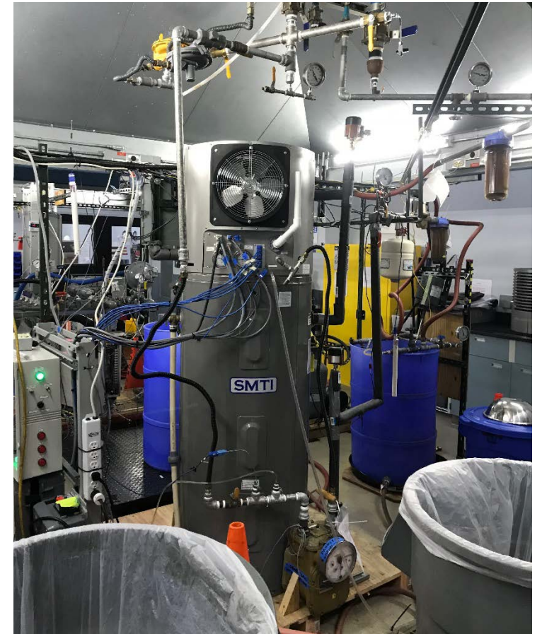
Photo of SCG Testing (Courtesy: SoCal Gas)
