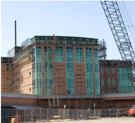
Commercial New Construction
