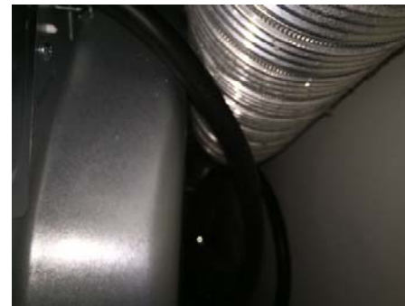
Image: Timothy's crushed dryer vent at home
