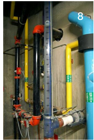
Greywater recycling system, Kiowa Co. Memorial Hospital, Greensburg, KS [NREL image]
