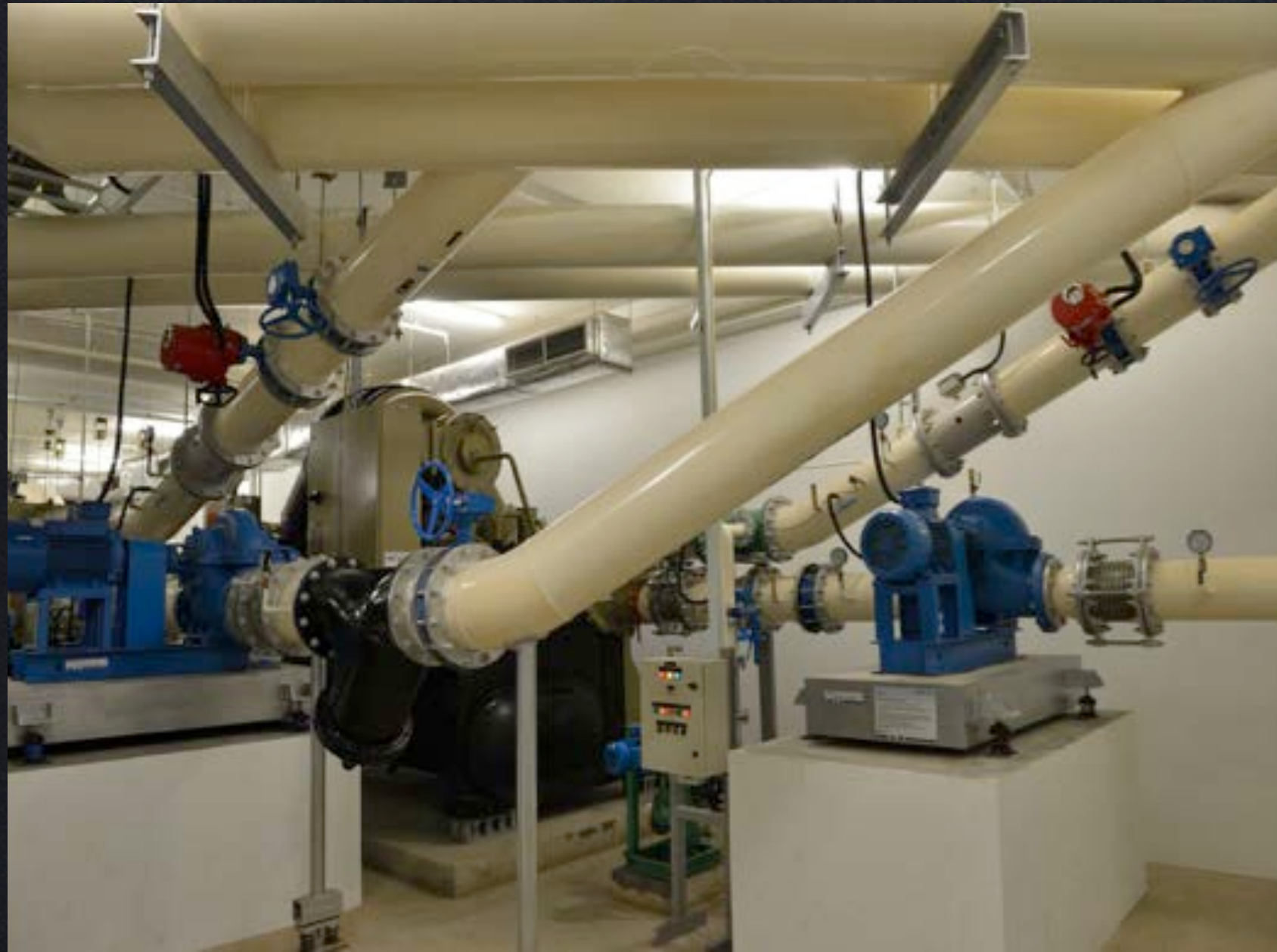
Big pipes, small pumps
