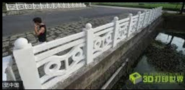
Chinese 3D-printed bridge girder and railing
