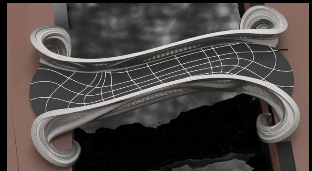
The artistic 3D-printed 12.5m stainless-steel bridge over Amsterdam's Oudezijds Achterburgwal canal
