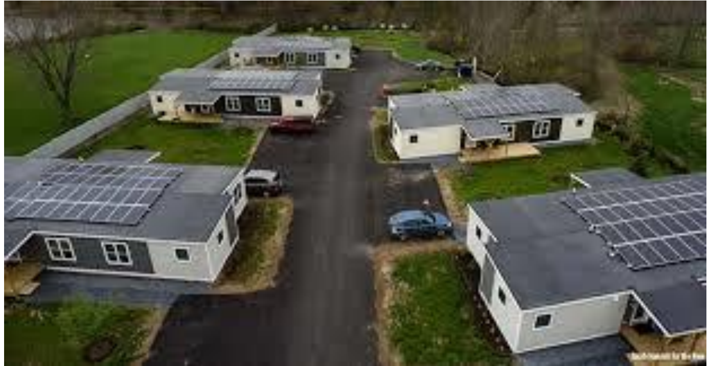
Zero-energy modular homes on McKnight Lane in Waltham, Vermont. Source: VHCB 2020b .
