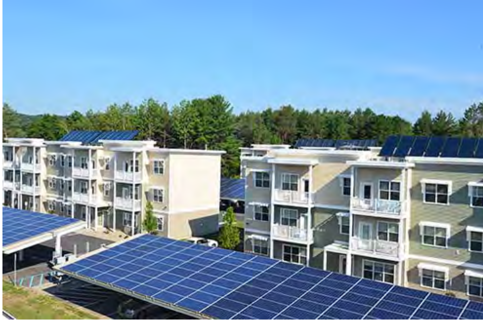
Figure 4. The low-rise NetZero Village in the New York Capital Region. Source: Goodell 2019.
