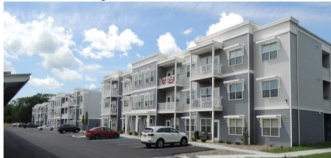
Figure 4. Solara Apartments, Rotterdam, NY – Imagery Credit: Photo Courtesy of Harris A. Sanders Architects, P.C., and Black Mountain Architecture.
