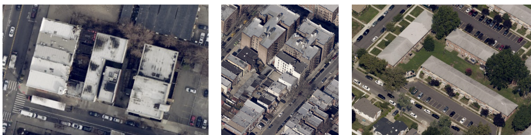
Figure 1: Example of multifamily buildings seen in orthogonal (left) vs. oblique (center and right) aerial imagery captured via low-altitude fixed-wing aircraft. Imagery source: Pictometry International Corp. Copyright © 2023. All Rights Reserved.
