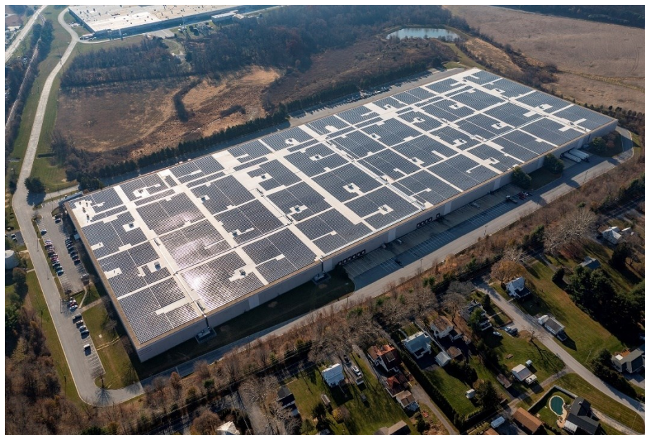
Figure 4. STAG Industrial’s 9.6-megawatt community solar installation in Hampstead, Maryland. Source: STAG Industrial.
