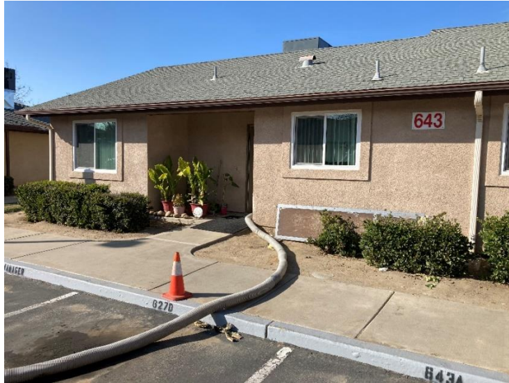
Figure 1. Apartment at Site 1 during attic insulation removal
