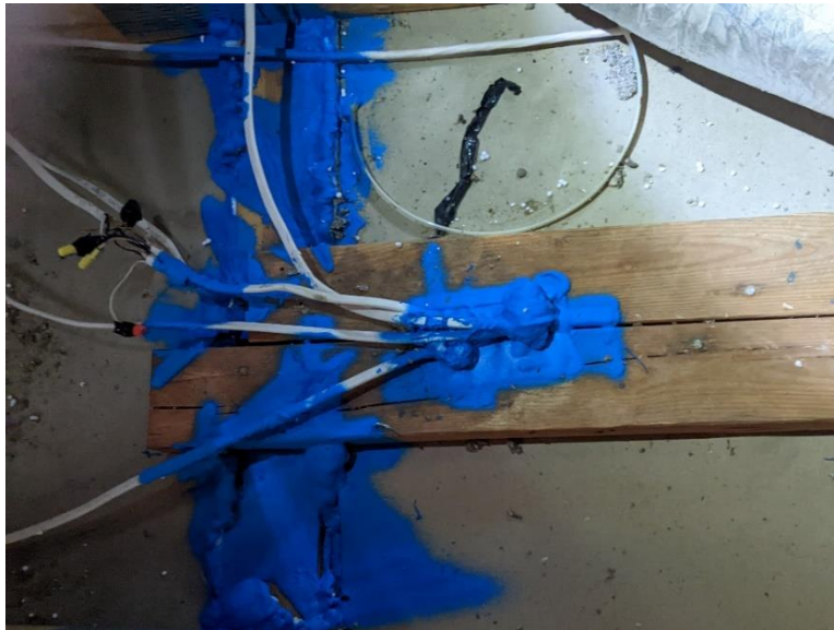
Figure 4. Photo of elastomeric seal product in attic
