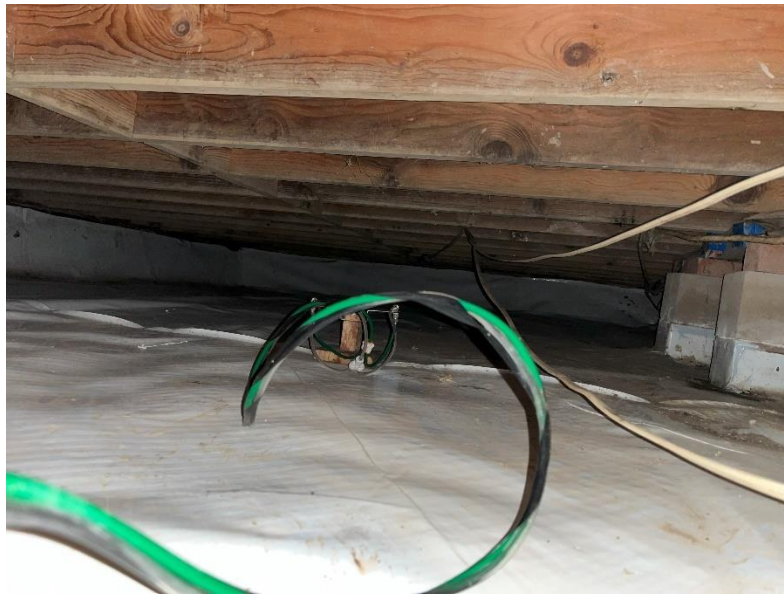
Figure 7. Photo of crawlspace sealed at Site 4
