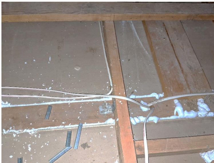
Figure 3. Photo of seals formed with can foam during manual sealing effort
