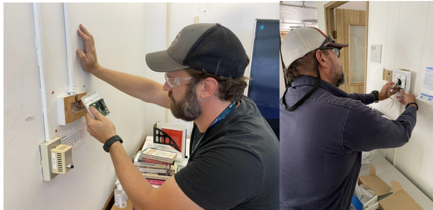
Figure 6. Images of ICs installing networked thermostats.
