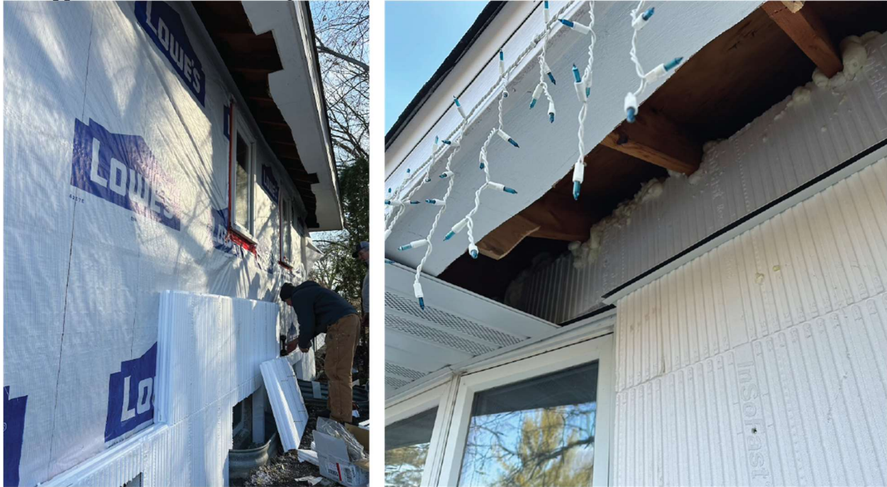
Figure 12. WRAP Installation in Progress (photo courtesy Paul Cole, SRC)
