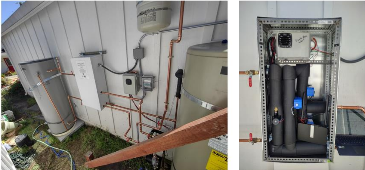
Figure 5. A photo of one of the LOCUS retrofits at Santa Rosa (left) and a close-up of the internal manifold of the LOCUS (right). The tank on the right side of the photo is the primary storage tank, and the tank on the left side is the added storage. Note that this photo was taken before pipes were insulated.
